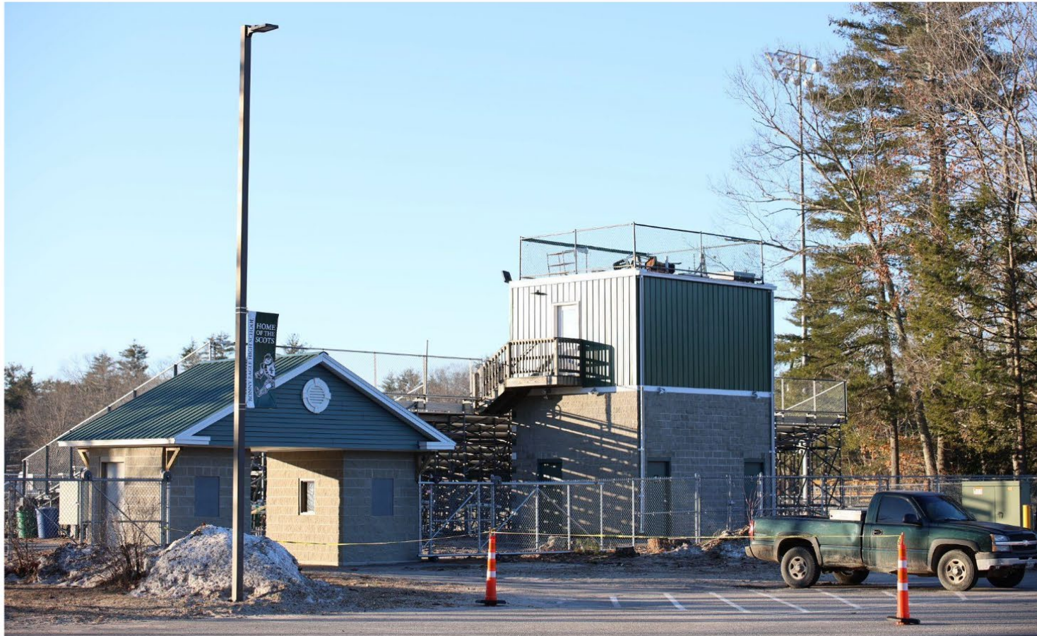
BEHS Stadium - Tree Demo at Press Box/Seating
