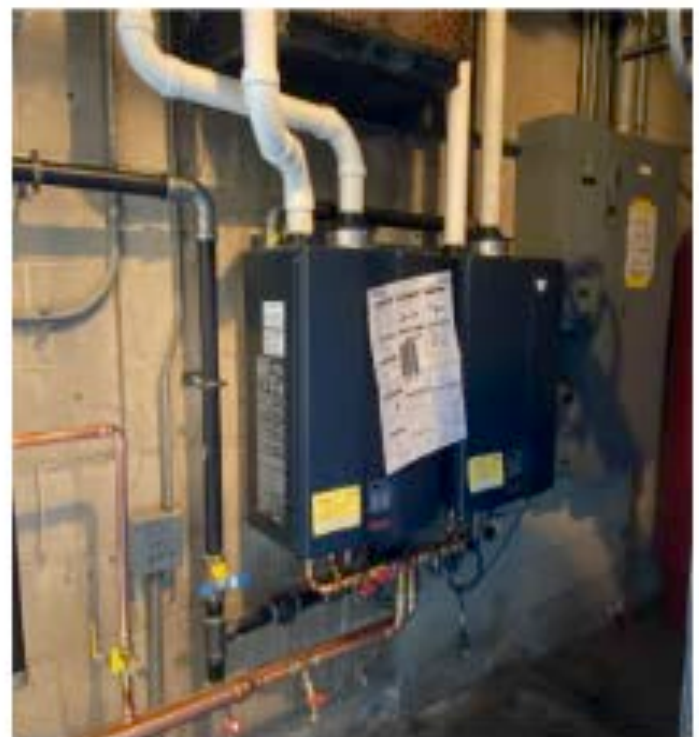
BEMS - LP Gas Hot Water Heater
